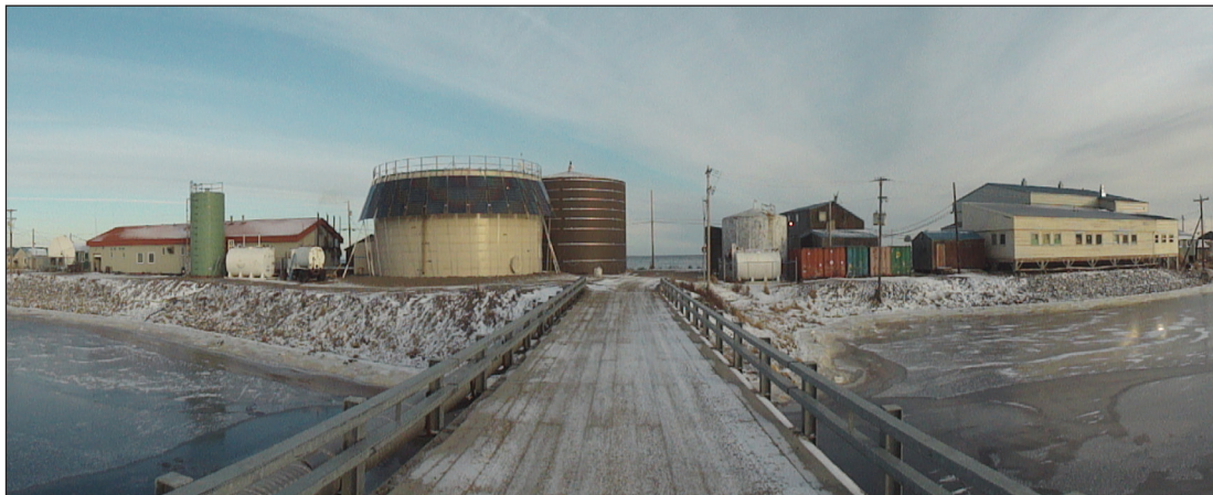
Solar panels provide power to the water treatment plant in the North West Arctic Borough community of Deering. Photo by Rob Bensin.
