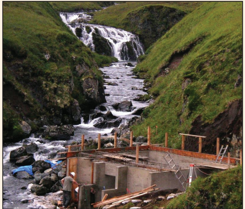
Humpback Creek during construction. Photo courtesy of Clay Koplín, CEC.
