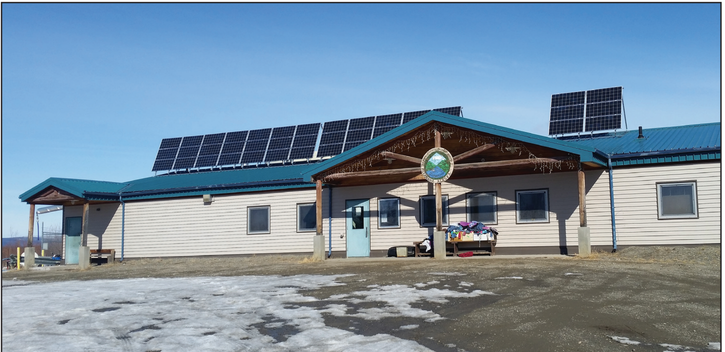
The City of Tanana’s washeteria uses solar PV, biomass, and diesel to heat the domestic hot water. Photo by Amanda Byrd/ACEP
