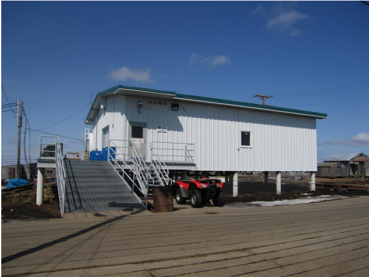
Figure 1: A diesel power plant in the village of Chefnak.
